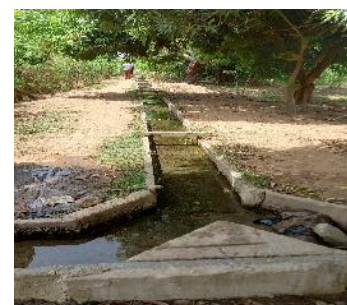
Canal derivation in reinforced concrete (primary and secondary canal)
