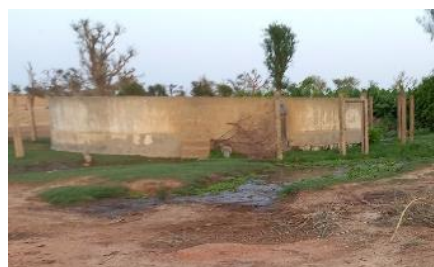
Water retention reservoir
