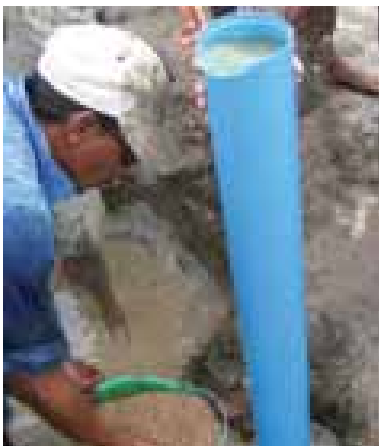
Pouring gravel in the borehole, water will overflow the pipe
