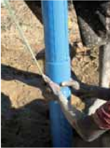
Use of rope during installation
