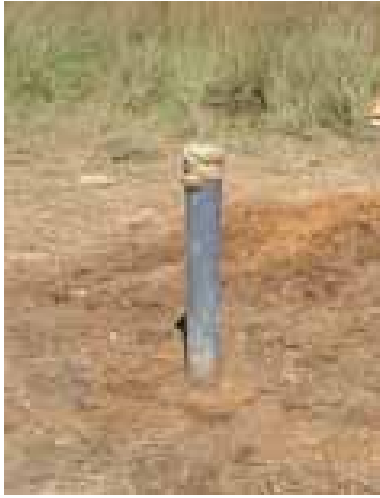
Backfilling has finished The top of the pipe is protected
