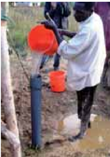
Flushing the well with water
