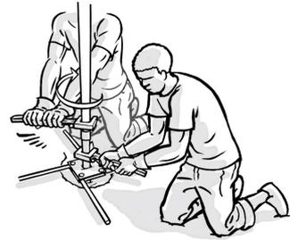
Take and log a sample of the drilled soil, every meter or every time before a new pipe is added. Take the soil sample from the upper part of the smaller mud pit.
