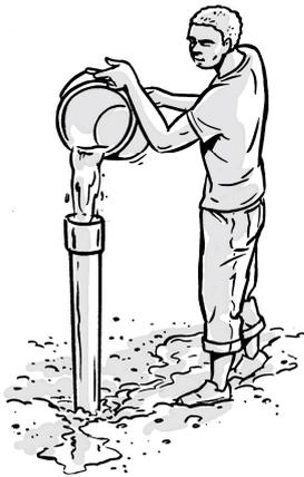
Drain the dirty water away from the mud pits. Pour clean water into the casing and allow dirty water to overflow the borehole until clean water comes out of the borehole.
