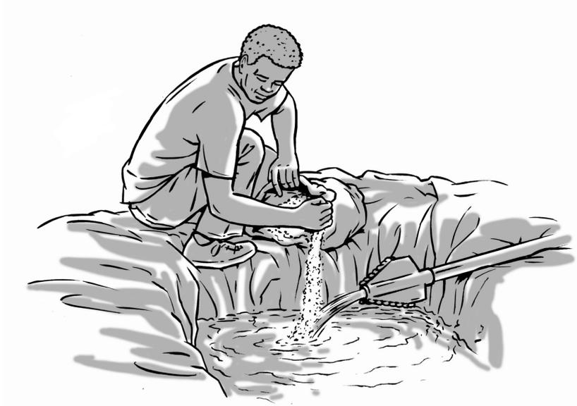
Set the valves on the pump so the water circulates within the mud pits (**circulation mode**). To redirect the water first open one valve, before closing the other to avoid damage to the pump.
