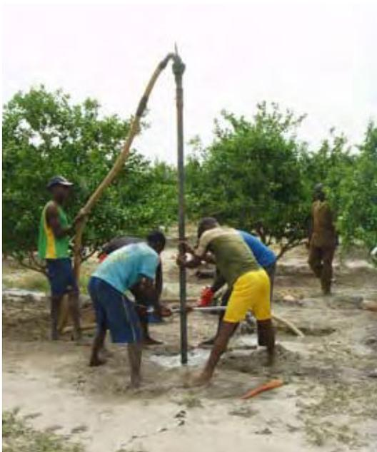
**JETTING** is based on water circulation and water pressure. As opposed to sludging, water is pumped down the drilling pipes. The large volume of water has an erosive effect at the bottom and the 'slurry' (water and cuttings) are transported up between the drill pipe and the borehole wall. A motor pump is used to achieve an adequate water flow. The drill pipe may simply have an open end, or a drill bit can be added and partial or full rotation of the drill pipe can be used.
