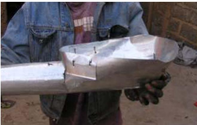
Photo 24: A pipe funnel can be made directly from the pipe. Photo 25: An example was made on Isaku house.
