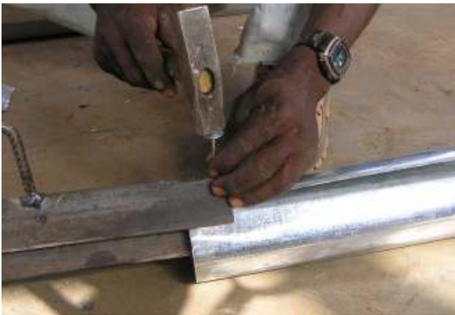
Photo 21: The ring of the perforator supports on the ground and perforating is easy.
