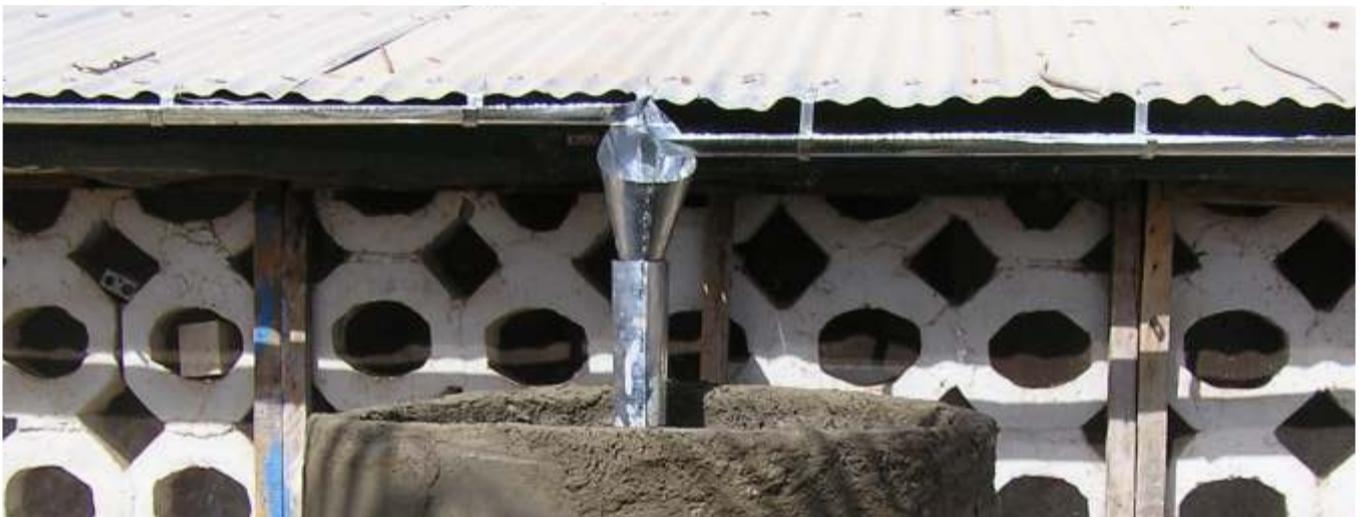
Photo 37 The first system installed with gutter which was too narrow.
