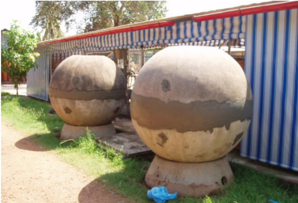
**Figure 11. Freshly constructed rainwater harvesting concrete tanks**
