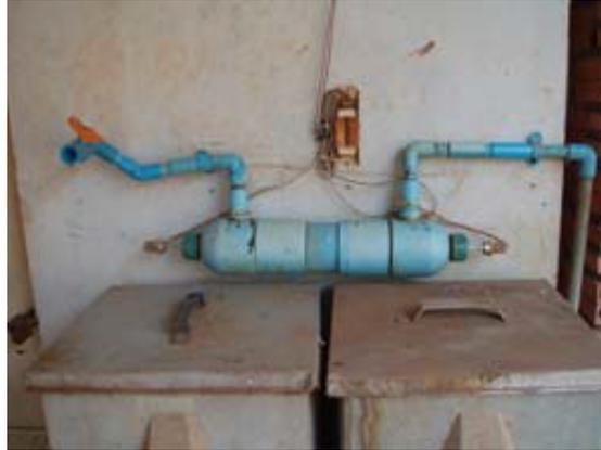
**Figure 33. UV treated rain water used in the *E. coli* test**
